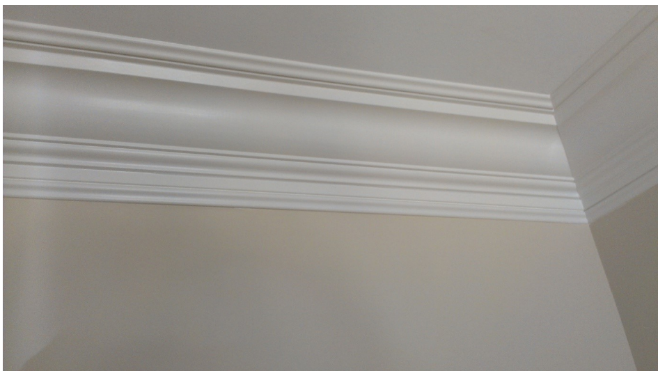
Crown Molding with double build-up
